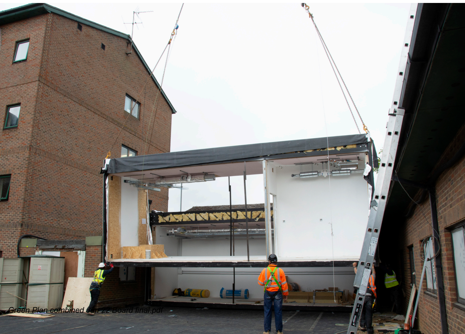
Construction of new emergency department
